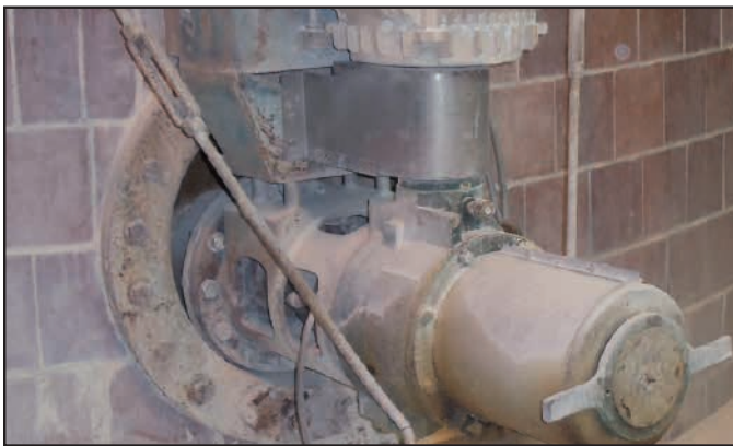
One of four slurry tank agitators installed with Inpro/Seal Air Mizers to eliminate product loss and decrease maintenance costs.
