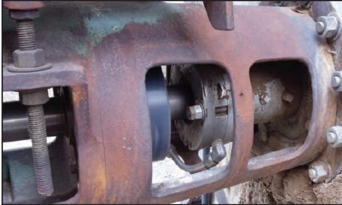
One of two split stainless steel Air Mizers installed on white liquor tank agitators.
